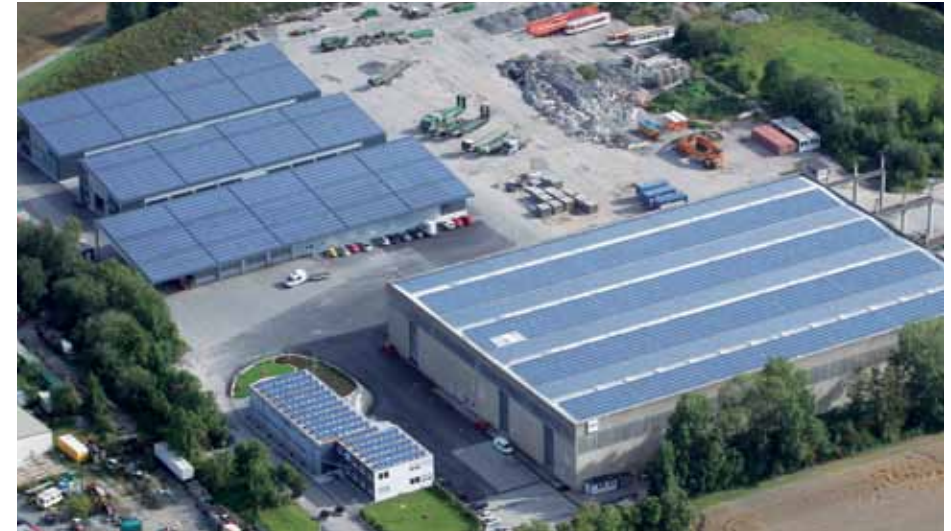
Novatech | Michelfeld-Erlin - Germany System: 1,4 MW | Solar fastener System
