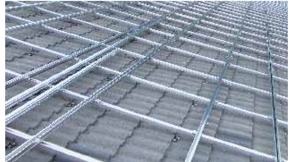
Elpo | Pfunders - Germany System: 484,65 kW | Vario 2 roof fastener with cross bracing
